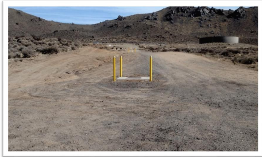
Photo 7. Koontz Lane below the water tank
